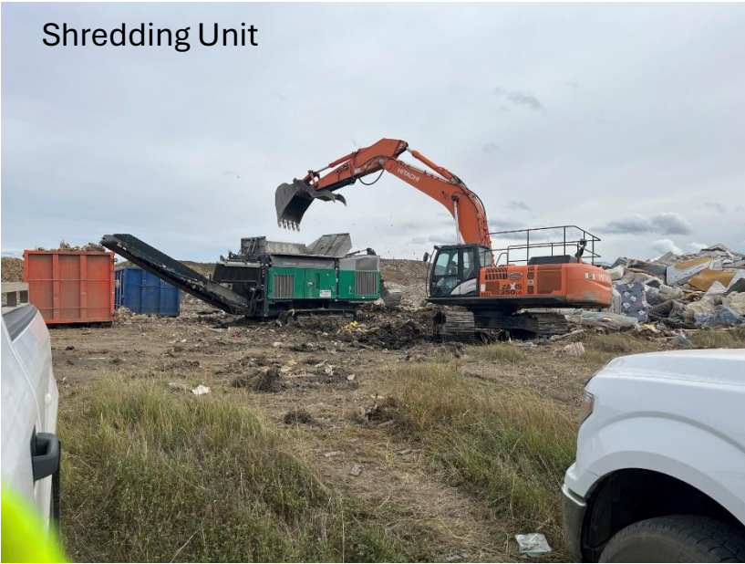
Mattress Pile Start
