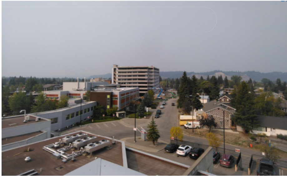
Parkade Construction Site
